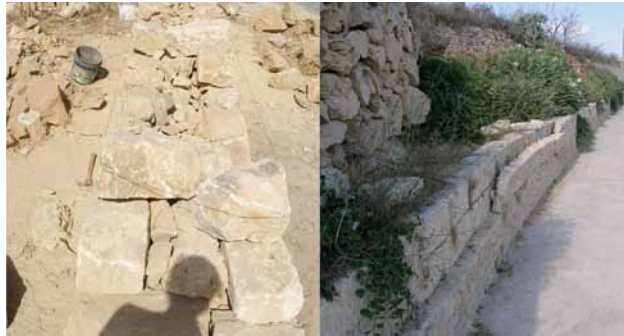
Figure 7: Left, a dry rubble wall under construction. Right, a false wall eroding away.
