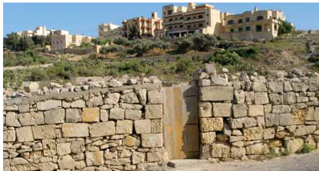
Figure 11: A wall with multiple layers of construction.
