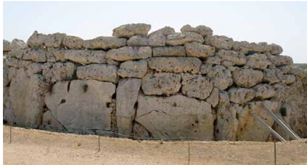
Figure 2: A wall of the Gigantija temple, the oldest standing structure in the world, built under the same principles as the terrace walls.
