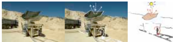
Figure 8: Saw for vertically cutting stone and the rails along which it drives in order to cut accurately.
