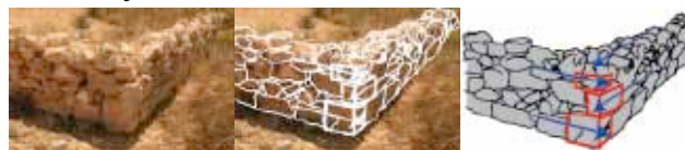
Figure 14: Strengthening the corner of a wall by a system of covering.
