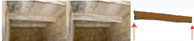
Figure 17: Lintels in the role of supporting elements that carry the roof.
