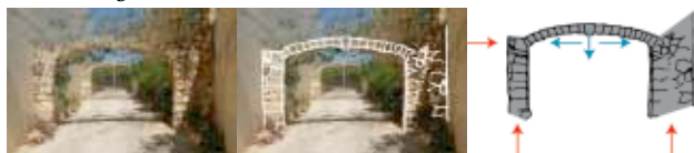
Figure 20: Extremely slender arch with a wide span built without the use of binding and the forces.
