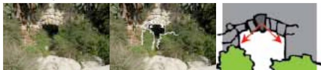
Figure 19: Typical example of the construction of an arch with a keystone.
